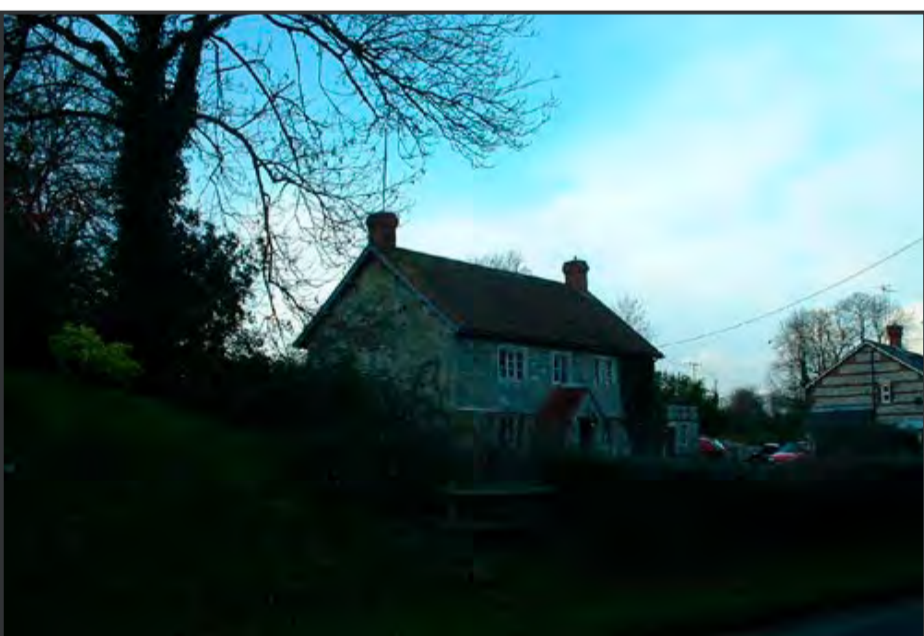
Stone and knapped flint chequerboarding on cottages is characteristic of the built environment
