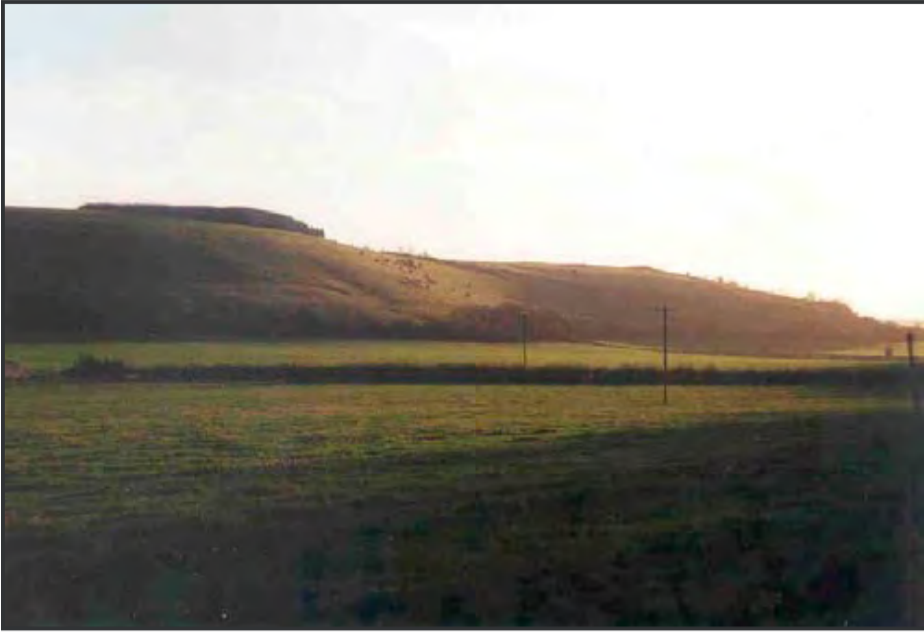
The vast escarpment looms over the adjacent terrace and forms dramatic shadows.
